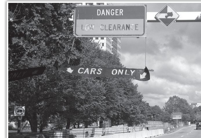
Boston's height-restrictors keep oversized trucks off parkways.
