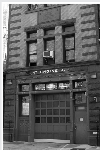
New York City firehouse dating from 1889 at 500 West 113 th Street.
