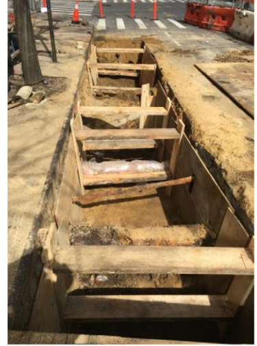
Excavation & sheeting for utility work
