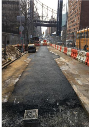
Temporary restoration for 20" water main
