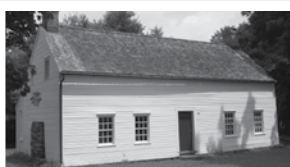
Photo by: Quasarjarvis
