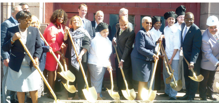
May 18th the Buffalo School District broke ground on the Emerson 2.0 School located at 75 West Huron Street, which is directly behind the current facility on Chippewa Avenue. It is expected to be open for students beginning September 2019.
