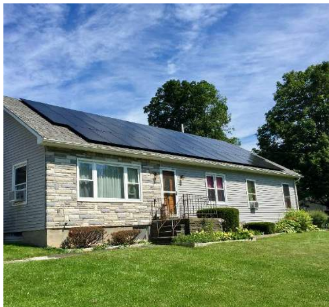
Image 16. Residential solar installation. Photo credit: Kasselman Solar.
