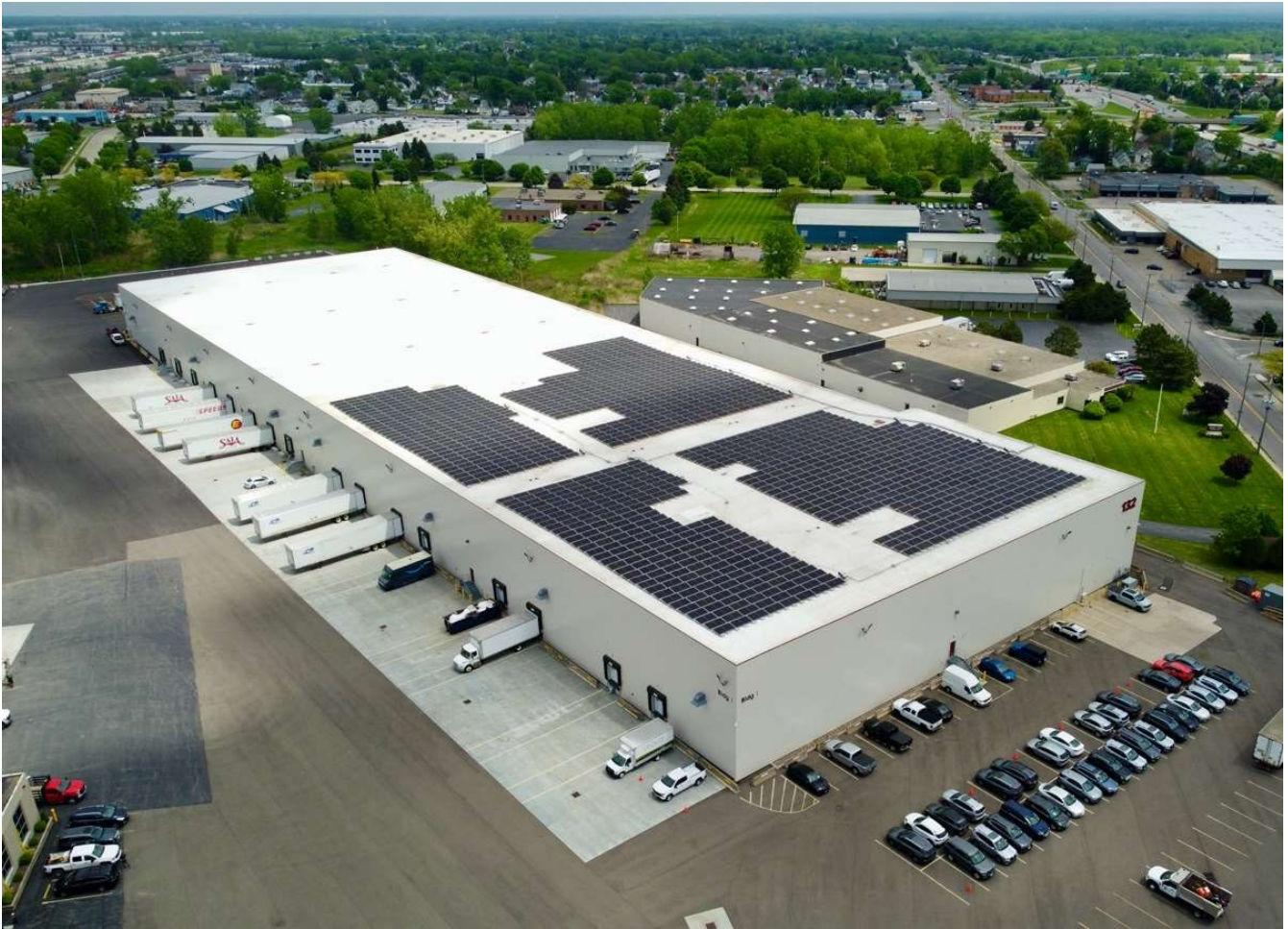
Image 11. Commercial rooftop solar installation in Buffalo, NY. Photo credit: Pinto Construction Services, Montante Solar.
