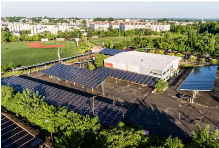
Image 10. Solar carport installation. Photo credit: Ecogy Energy.
