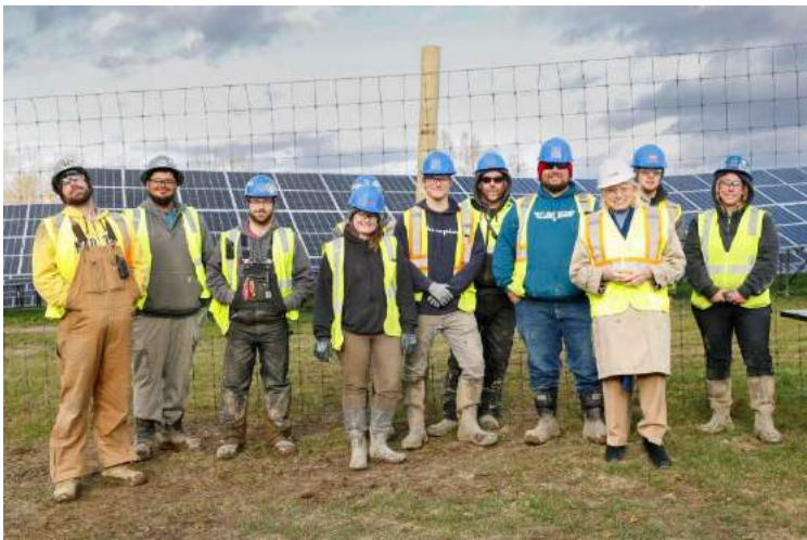
Image 7. Upstate community solar installation crew. Photo credit: New Leaf Energy.
